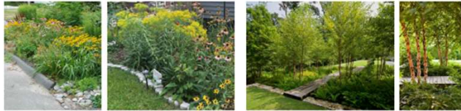
① Rain gardens - SuDS that capture rainfall before it enters the piped network and allows it to infiltrate into the ground.
