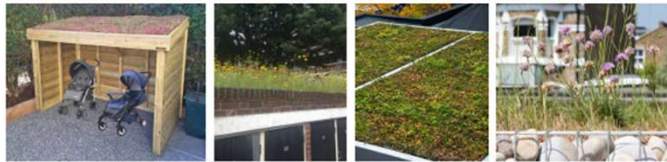
③ New buggy stores and bin stores with green roofs for water management and wildlife benefit.
